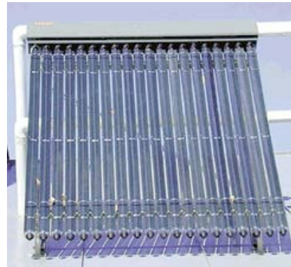
Below: A Thermomax evacuated tube collector.
