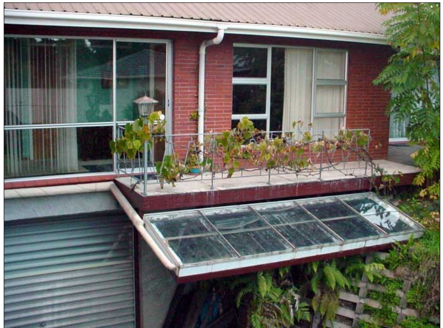
Almost 30 years old and still working! A well made home-built solar water heater can last as long as a commercial product.
